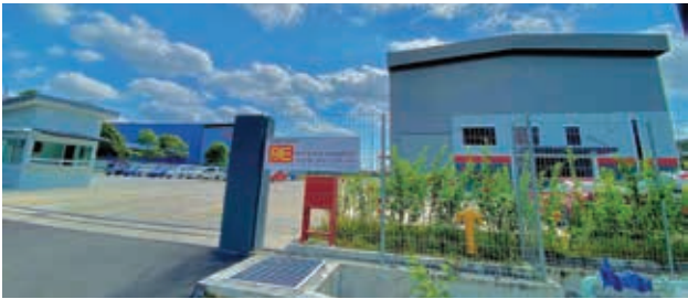
(Our newly constructed fabrication facility in Pengerang, Johore, Malaysia)
