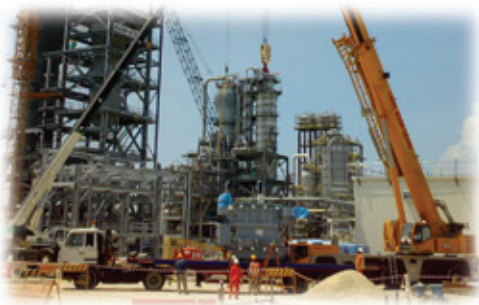
Installation of Transformer
